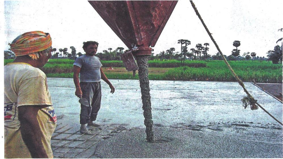
Raft foundation being laid using dynamic concrete for a commercial complex at Vizianagaram. (Right) Self-compacting concrete being poured for a concrete slab of an industrial unit in Visakhapatnam district. -- PHOTO: BY ARRANGEMENT
