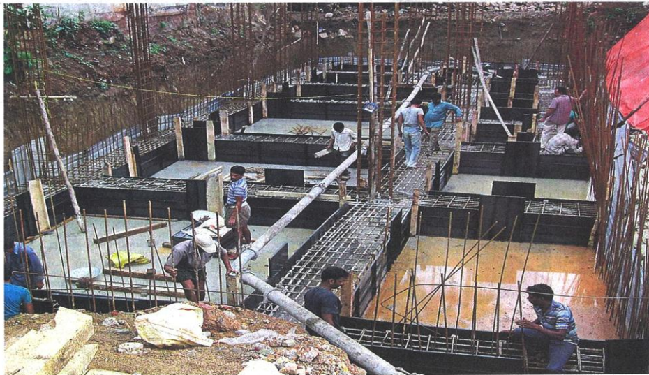
Raft foundation being laid using dynamic concrete for a commercial complex at Vizianagaram. (Right) Self-compacting concrete being poured for a concrete slab of an industrial unit in Visakhapatnam district. -- PHOTO: BY ARRANGEMENT
