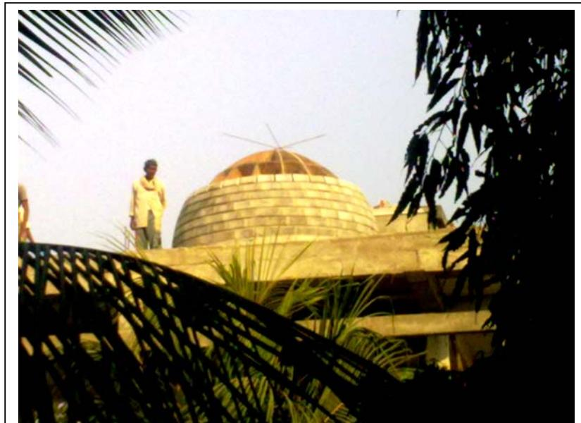
9-ft dia dome with FaL-G interlocking blocks as a demonstration structure
