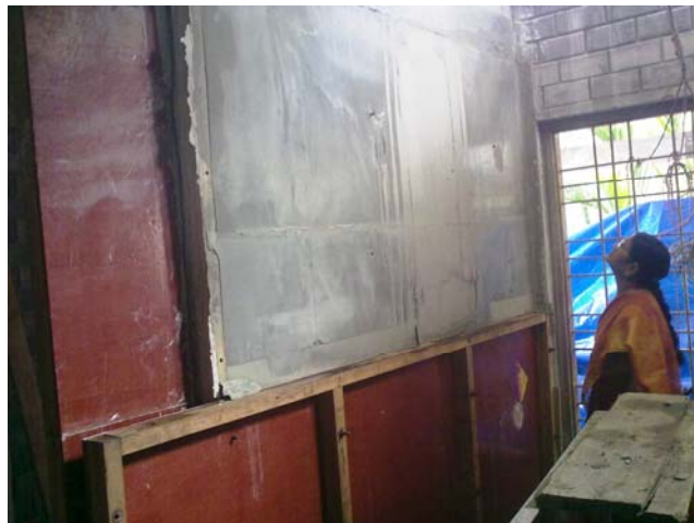
Cast in-situ wall with NAC : De-shuttered partially
