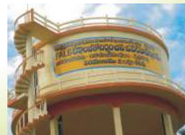
Overhead water tank built by Pantchayat Raj Dept., Govt. of A.P. using FaL-G concrete (Nagayalanka, Krishna Dist., A.P., India)
