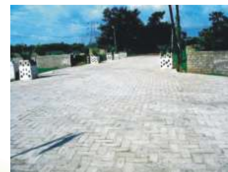
High strength FaL-G (30 MPa) blocks used in laying khadanza (brick-on-edge) pavement (entrance of INSWAREB Building Centre, Visakhapatnam, A.P)
