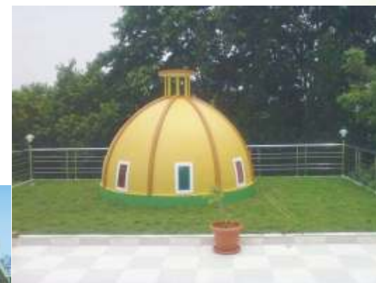
Dome with NAC at eastern face lift of FaL-G Mansion
