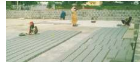
Casting of FaL-G bricks in the lines of clay bricks
