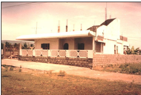
FaL-G Mansion 1991-slab with FaL-G concrete in lime route without using even a gram of cement
