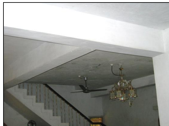
Tie beams in FaL-G concrete slab
