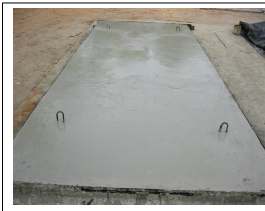
Precast roofing panels (5 x 2 mtr) cast at GVP Medical College Project, Visakhapatnam, India, being lift on 7 th day with 50 MPa strength.
