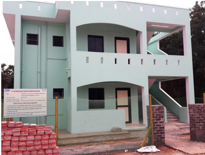
Demo Building at Deepanjali Nagar, NTPC Simhadri Power Project, Paravada, using Nano Concrete aggregate (NACA) as total replacement to natural stone aggregate.
