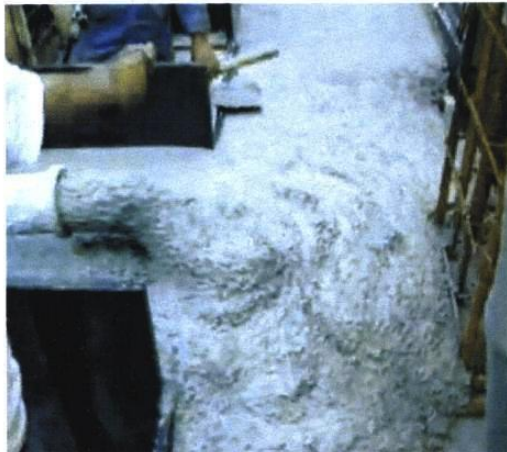
Pumping of Dynamic Concrete
