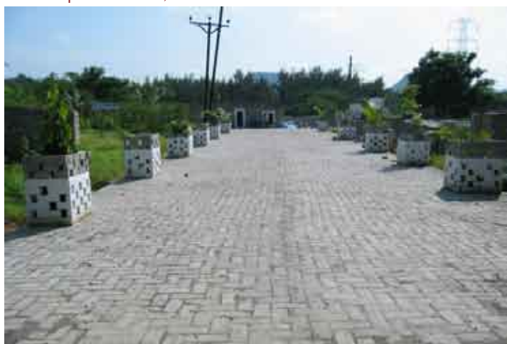
Pavement constructed with FaL-G bricks in Parawada, Visakhapatnam District, Andhra Pradesh
