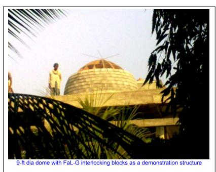
Another 9 ft dia dome was built wth FaL-G interlocking blocks over the stair case block on the western elevation.
