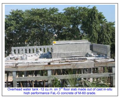
The mortar and concretes have been prepared containing 50 to 75% fly ash as cement replacement. Many of the beams and columns, including the overhead water tank of 12 cu.m capacity, have been cast with self-leveling concrete rendering M-50 to M-60 grade.
