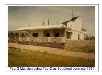
First floor onwards to the top, including 6 cu.m. overhead water tank, the structure was built with Portland:FaL-G in the ratio of 30:70; using the same as mortar, PCC and RCC.
