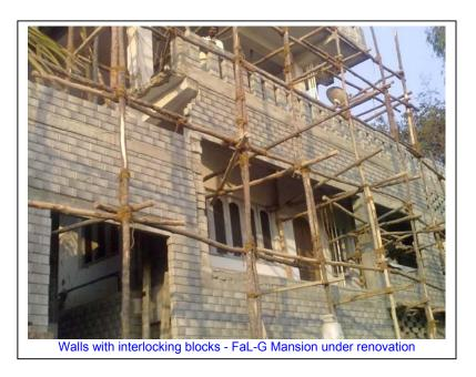
In the refurbishing activity, the basic structure that has put on 20 years of life, made of FaL-G concrete, was not disturbed. During the reorientation of rooms and partitions, walls have been made of interlocking blocks containing 75% fly ash in the cementitious mix.
