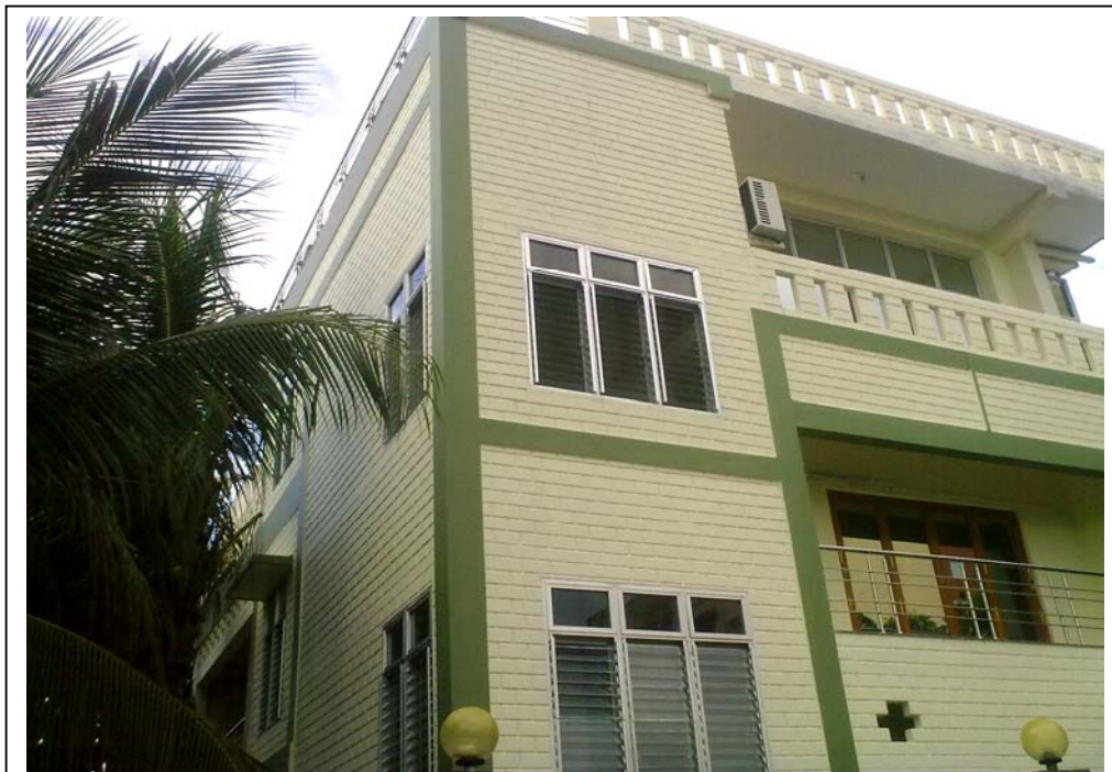
South-side elevation – outer wall is built of FaL-G interlocking blocks – no plastering done.
