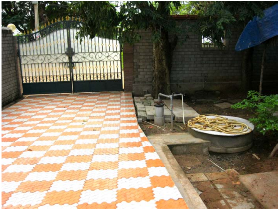
North-east gate – The main entrance; Rainwater harvesting pit is on right side.
