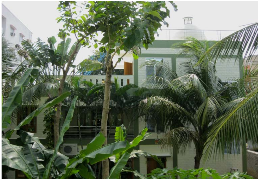
Western Elevation; Dome on 3 rd floor is made up of FaL-G interlocking blocks
