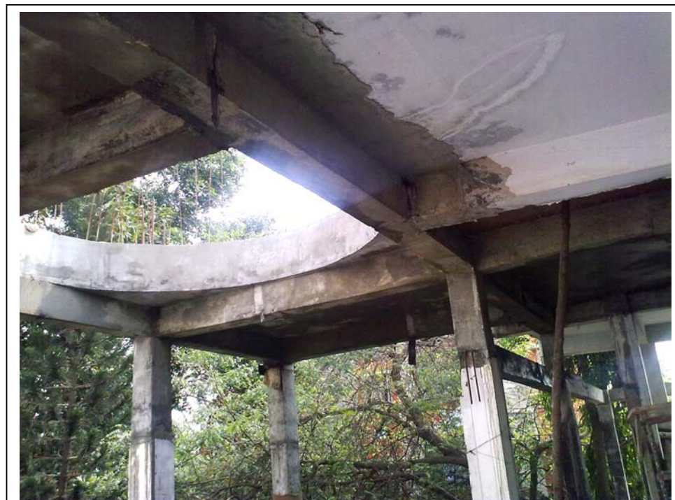
Starter for dome on 2 nd floor; extending 1 st floor columns to 2 nd floor – Eastern side face-lift
