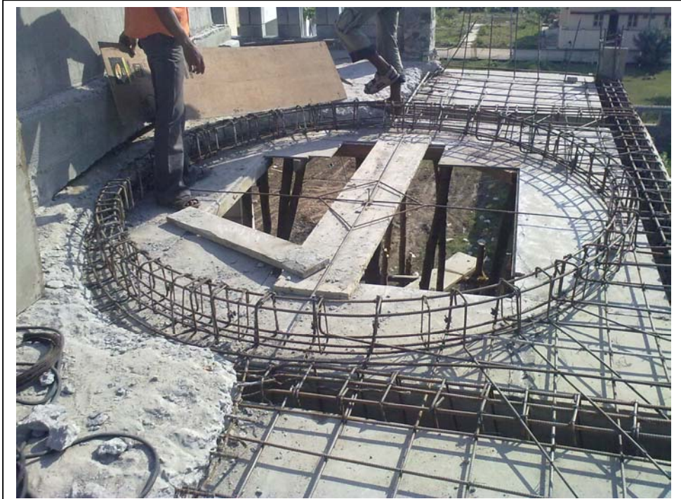
Reinforcement for starter beam to Western dome with FaL-G interlocking bricks; on third
