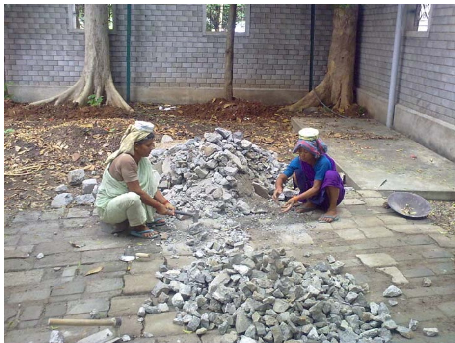
Almost all the demolished brick and concrete is put back into concrete for non-critical structural applications
