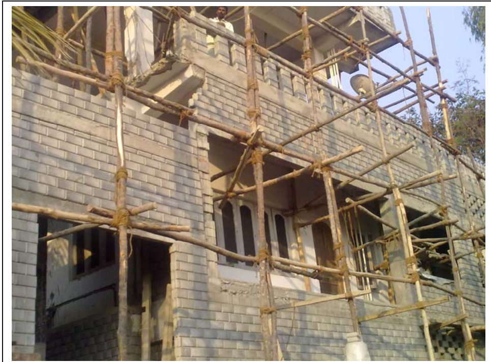
Walls with 4.5" interlocking blocks – Southern side face-lift
