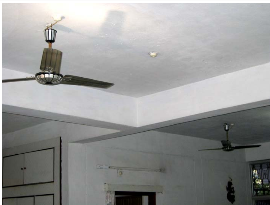
15 ft tie beam resting on another 15 ft beam to the slab of ground floor (1991); cast with concrete made of FaL-G in lime route, having not even one gm of OPC.
