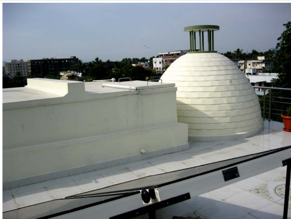
Third Floor: 12 m 3 water tank; dome made of interlocking blocks on western elevation.
