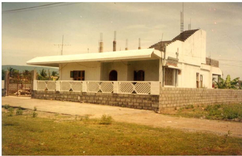
The first phase of FaL-G Mansion; Ground Floor slab together with beams was cast in 1991 totally with FaL-G concrete in lime route, having not even a gram of OPC.
