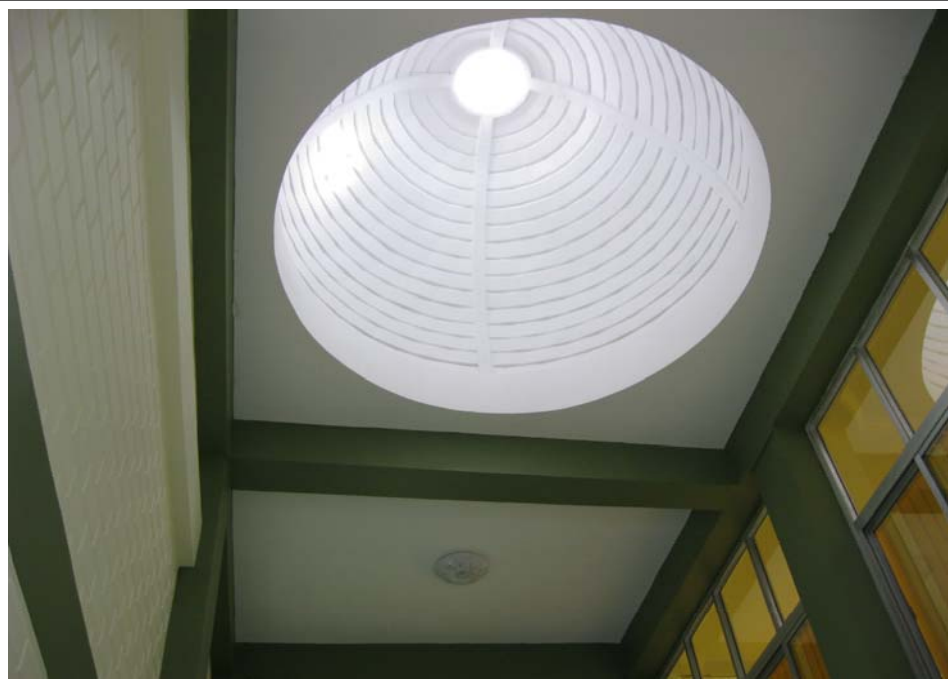
Dome with Interlocking blocks – bottom-view from the second floor
