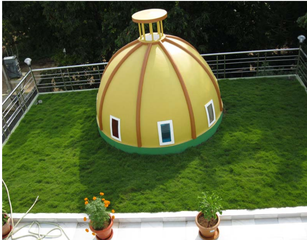
Second floor: Dome made of No-Aggregate Concrete (NAC) – Lawn is grown on the same floor, demonstrating the water-imperviousness of the slab.
